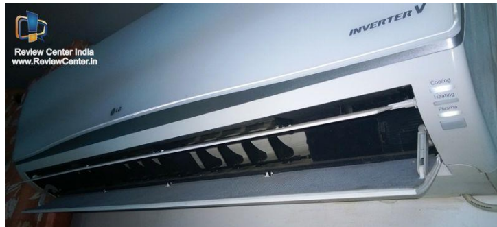
Figure 5. Blades that control airflow direction by motor swing.
